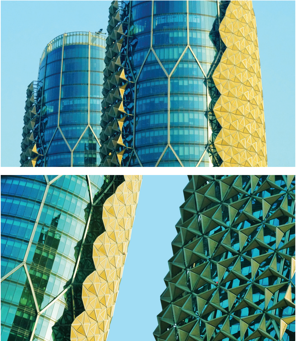
Figure 1: Exterior of Al Bahar Towers in Abu Dhabi
