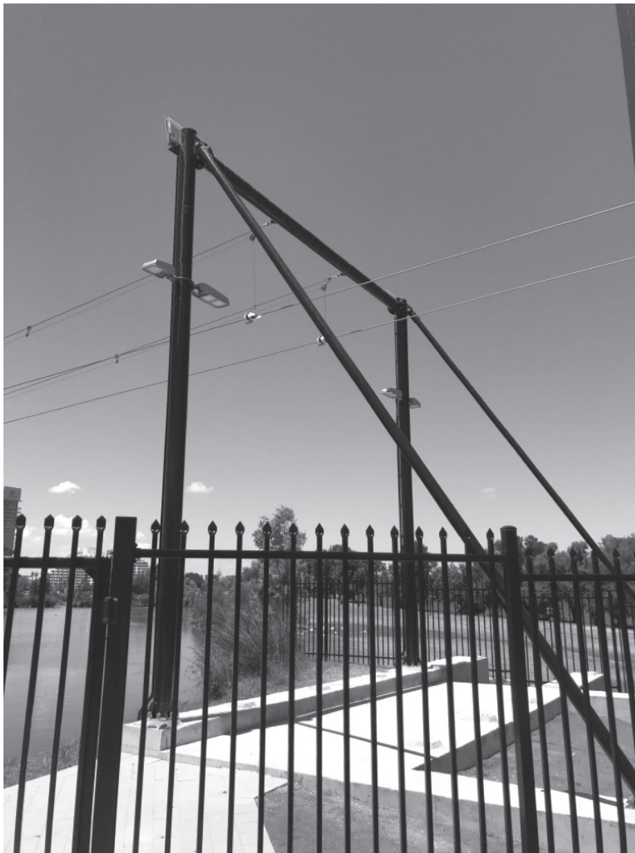
Existing flying fox frame, riverbank side
