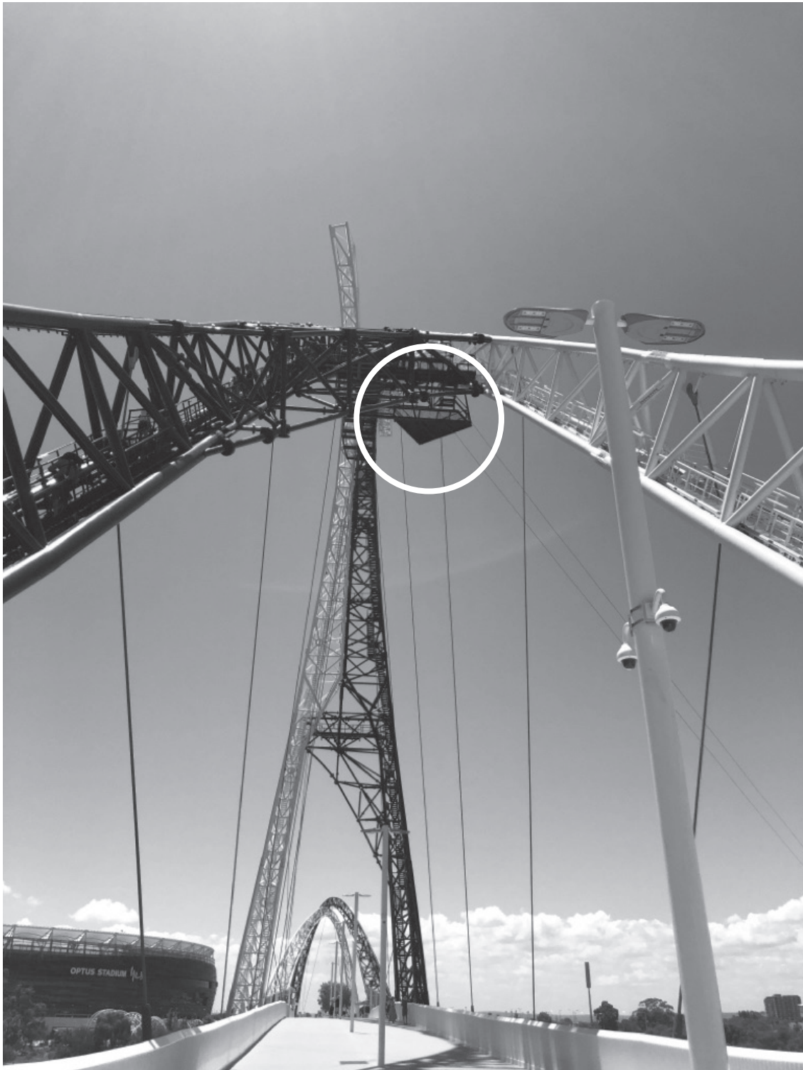
Existing flying fox frame, bridge side
